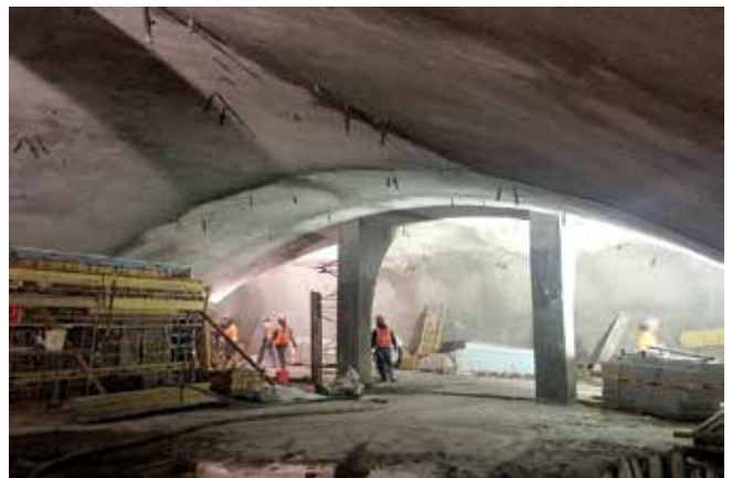
Fig. 7: Upper-level arch of TT#1 structure, tunnel, and cross-passage interface (opposite view)
