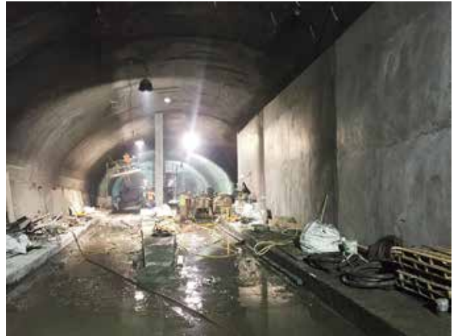
Fig. 12: Finished GCT 1/2 arch with rod finish. Walls were rubber float finished
