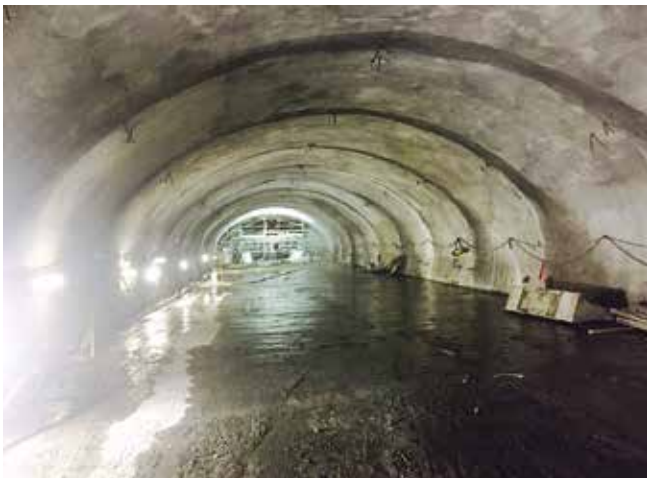
Fig. 11: Finished access Tunnel 1 arch with rubber float finish
