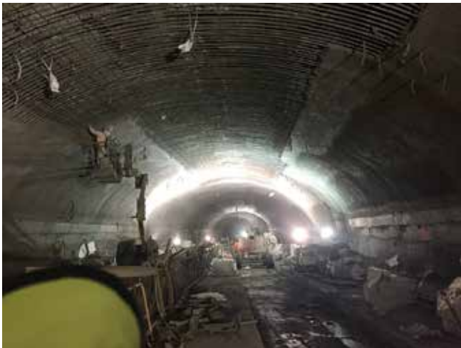
Fig. 10: Installation of GCT 1/2 arch with rod finish, working from boom lifts
