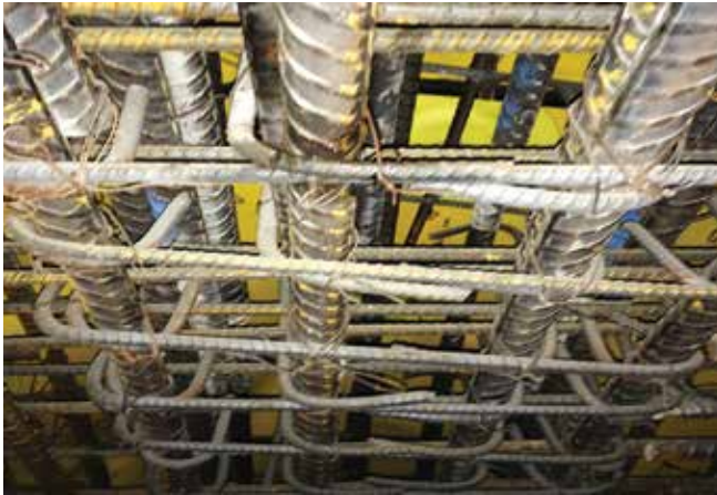
Fig. 5: Reinforced beam section in upper-level arch of TT#1 structure
