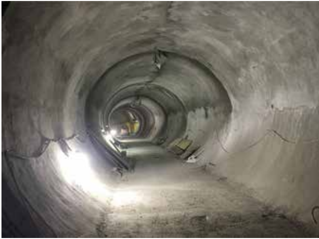
Fig. 9: Completed tunnel section
