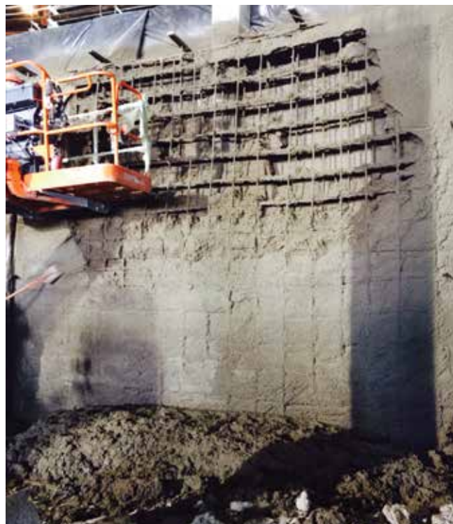
Fig 1: Moments after a potentially dangerous collapse of plastic material caused by stacking a wall too quickly
