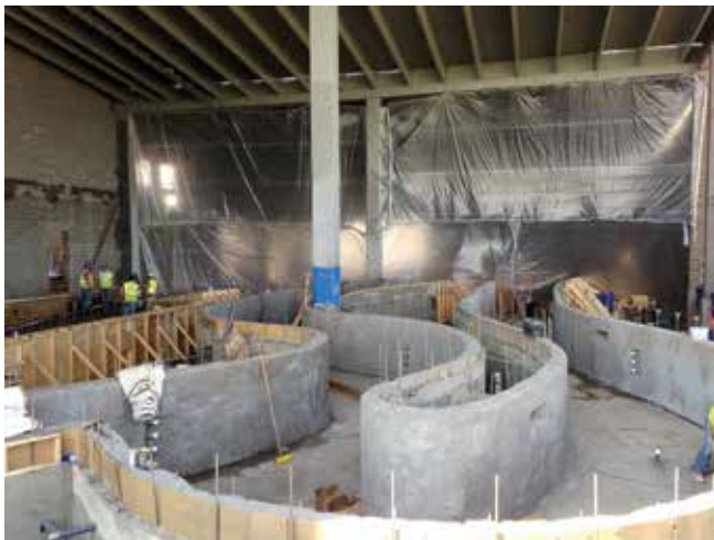
Fig. 1: First section of lazy river placed
