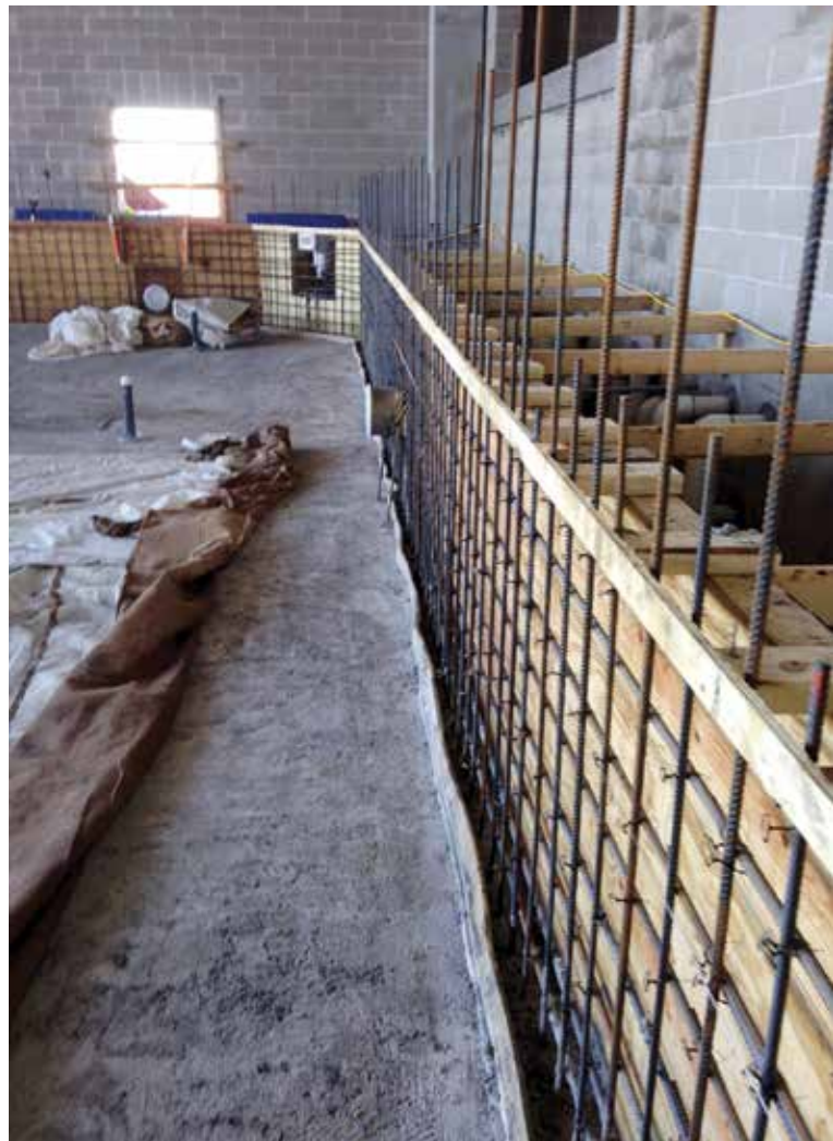
Fig. 3: Leisure pool ready for shotcrete application
