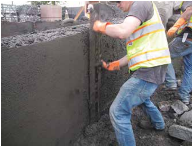
Fig. 16: Trimming shotcrete to shooting wires with cutting screed (rod)
