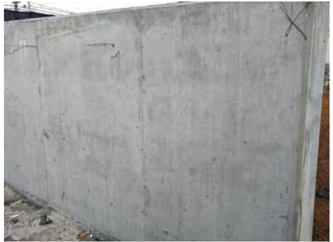
Fig. 18: Stripped face of L-shaped wall is defect-free
