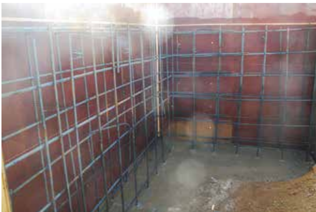
Fig. 14: Formwork and reinforcing bar for L-shaped wall
