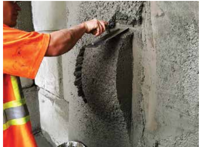
Fig. 8: Cutting and trimming natural fiber mixture (WNF) with no sagging or sloughing
