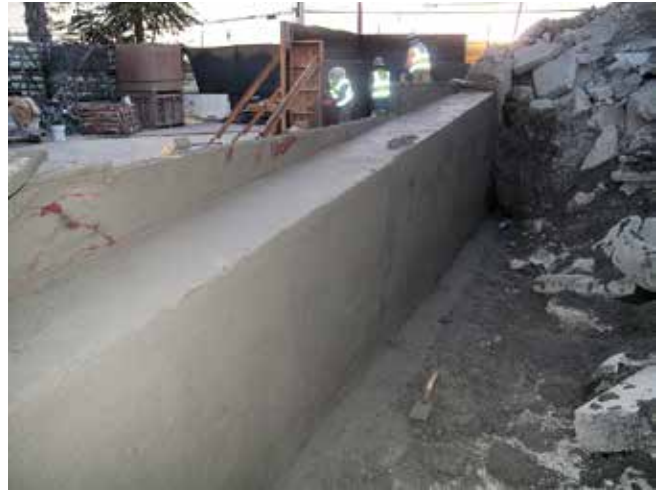
Fig. 17: View of finished straight wall
