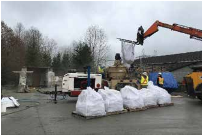
Fig. 2: Prepackaged dry shotcrete materials discharging into pan mixer
