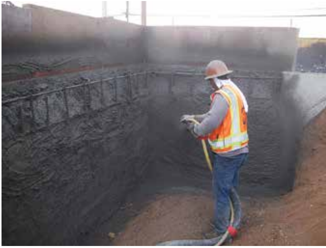
Fig. 15: Bench-gun shooting L-shaped wall
