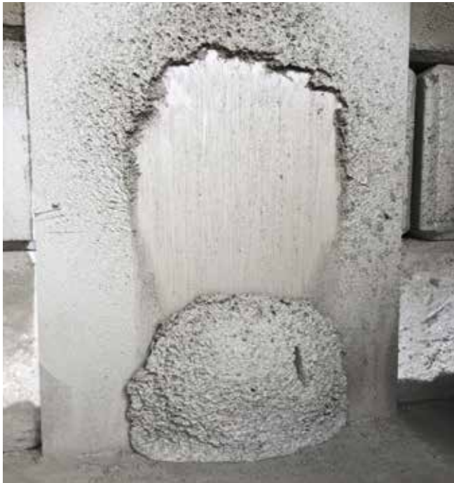
Fig. 6: Synthetic fiber mixture (WSF) sloughed off plywood panel after being disturbed by cutting
