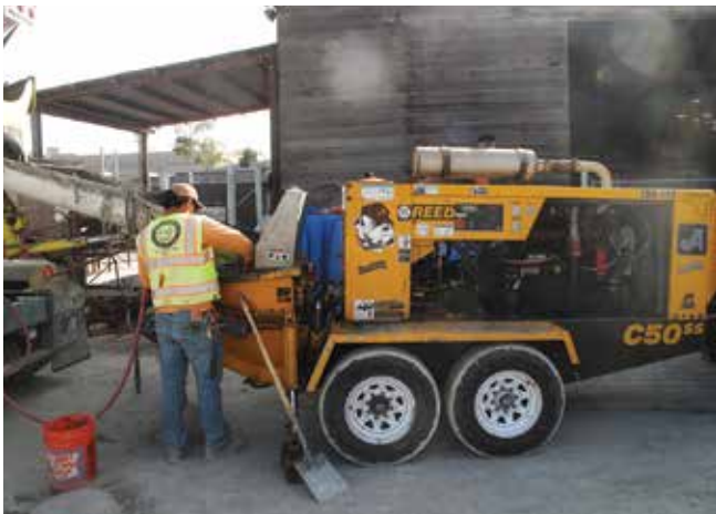
Fig. 13: Reed C50 pump used to pump wet-mix process shotcrete
