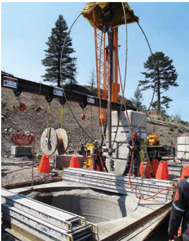
Fig. 2: Lowering the egg into shaft
