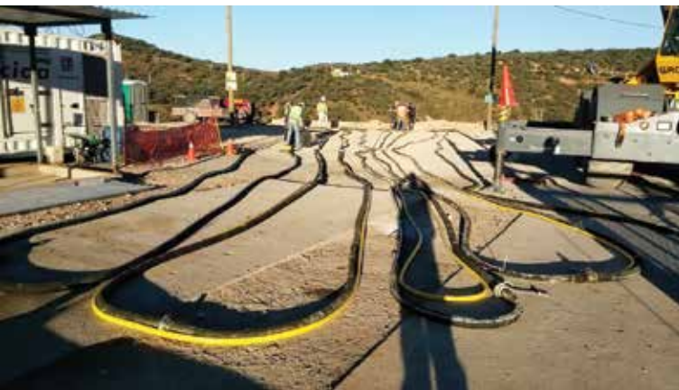
Fig. 1: Hoses before lining
