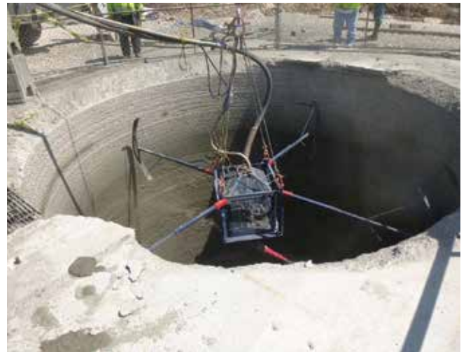
Fig. 3: Shaft lining with the spider
