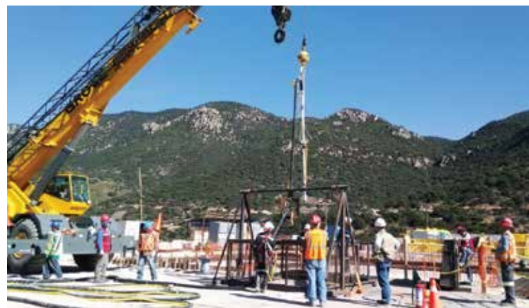
Fig. 4: Crane over the shaft
