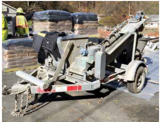
An auger-type pre-dampener used in dry-mix process refractory installations
