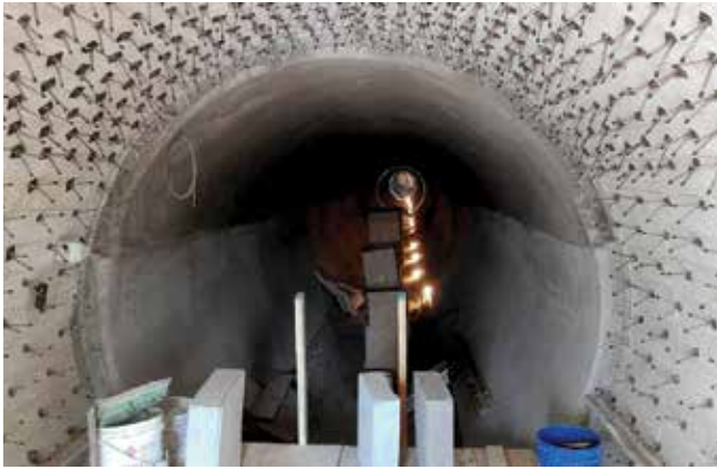
Refractory-lined 0.25 mile (0.4 km) long tunnel was placed with shotcrete
