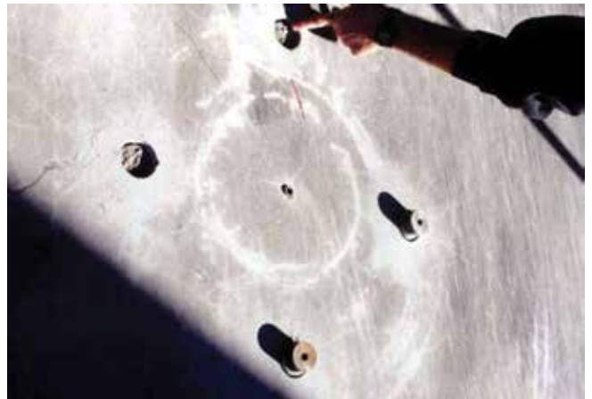
Fig. 4: Field testing according to ASTM C1583. Tensile bond pulloff conducted on repair using a silica fume shotcrete overlay. Setting acceptable values would be influenced by site conditions, especially the integrity of the substrate
