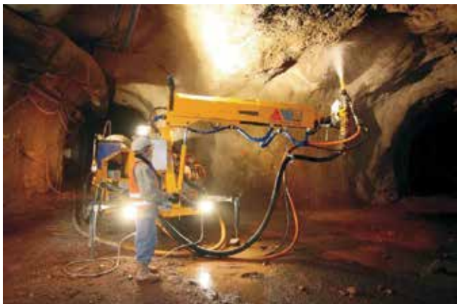
Fig. 8: Remote control wet-mix FRS ground support in mine in North America
