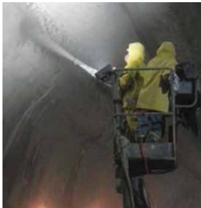
Fig. 2: Application of macro-synthetic fiber shotcrete in the Billy Bishop Pedestrian Tunnel 5
