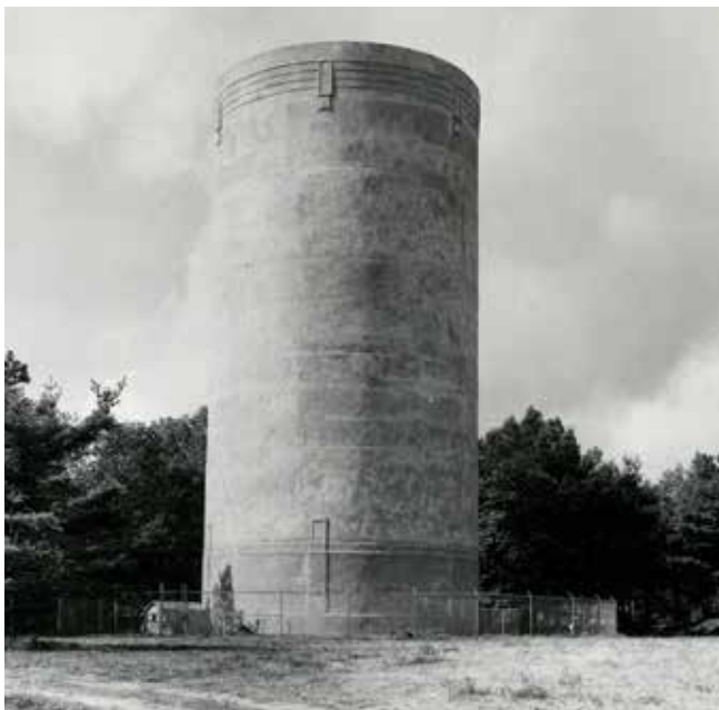
Fig. 1: Early prestressed shotcrete storage tank—circa 1936—in continuous maintenance-free service for more than 70 years
