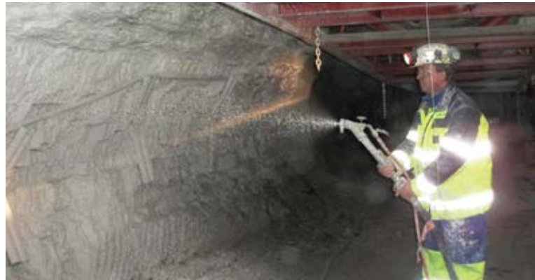
Fig. 4: Squeeze pump underground spraying
