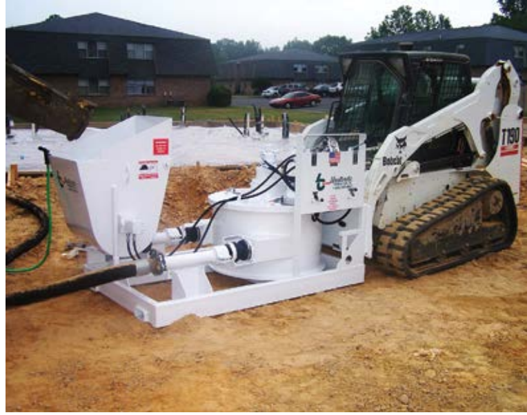
Fig. 2: Squeeze pump foundation pouring
