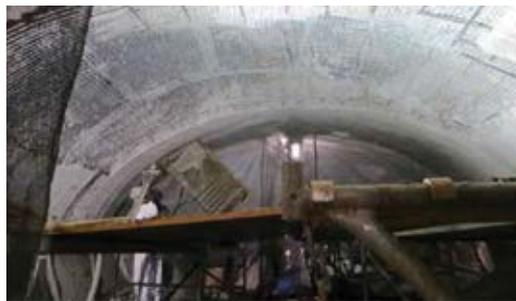
*Fig. 2: The STM engineering team identified approximately 6540 ft<sup>2</sup> (600 m<sup>2</sup>) of overhead area requiring removal and replacement, most of which ranged in thickness from 18 to 36 in. (450 to 900 mm)*
