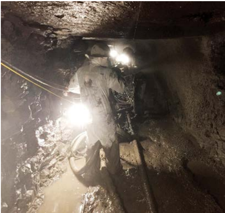
Working in confined spaces merits its own considerations and safety precautions
