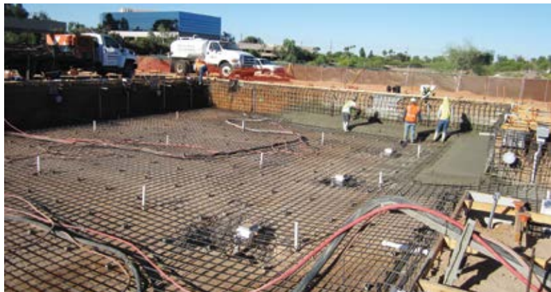
Fig. 2: The shotcrete (wet-mix process) floor being installed first
