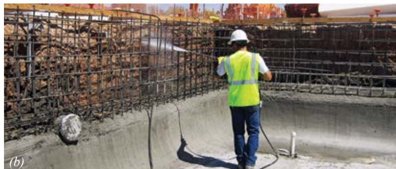
Fig. 8(a) and (b): Construction joints being prepared
