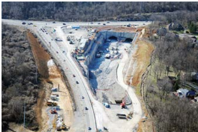
Fig. 4: Gene Snyder Freeway entrance construction site
