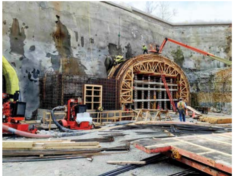
Fig. 8: Formwork for tunnel entrance
