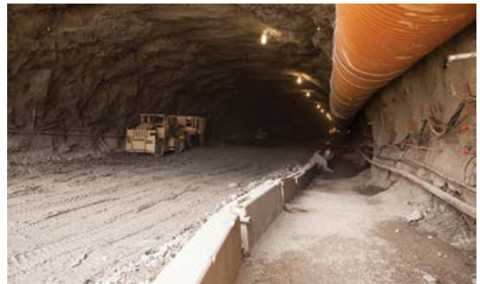
Fig. 5: 196,000 yd 3 (150,000 m 3 ) of rock and dirt excavated for the tunnel
