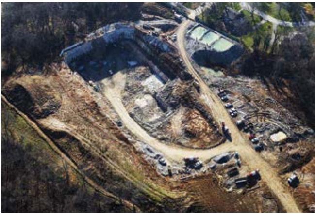
Fig. 6: Construction access from the north portal also needed to be created
