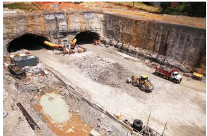
Fig. 7: Ventilation tubes exiting the south portal during construction
