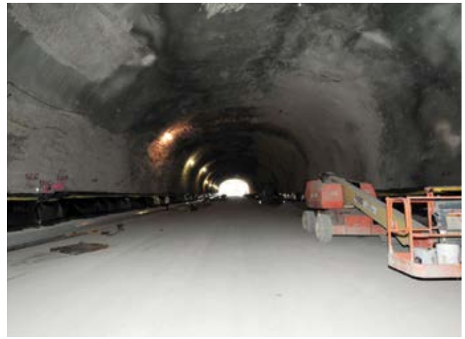
Fig. 10: Smoothed finish after hand nozzling
