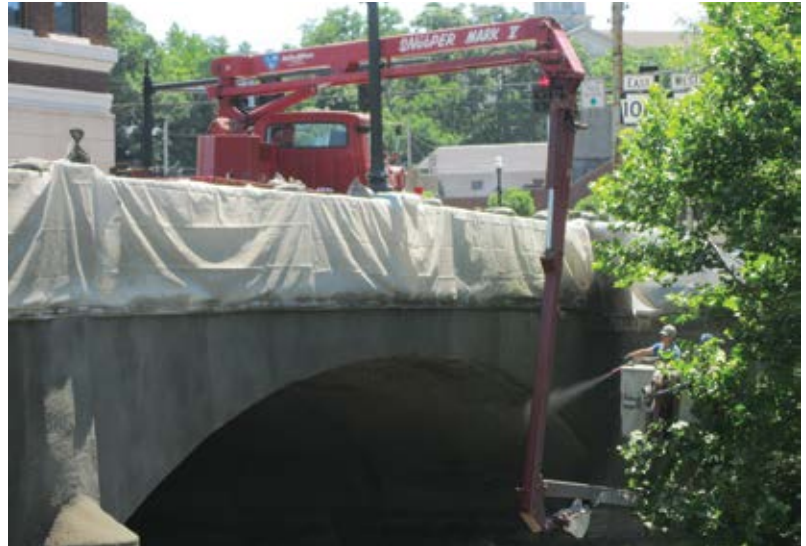
Fig. 2: On two-lane bridges like the one pictured above, lane closures are often necessary to provide access to the work
