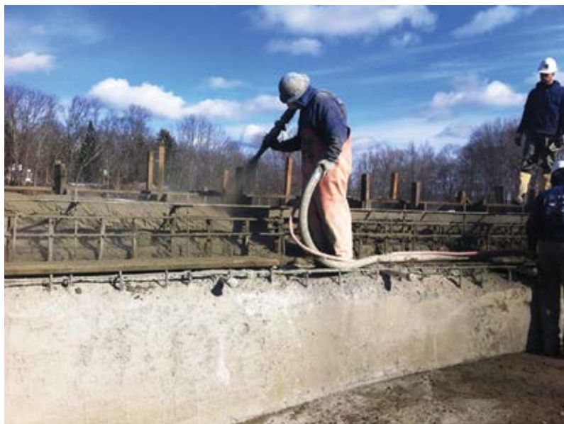
Fig. 1: ACI Certified Nozzleman applying wet-mix shotcrete
