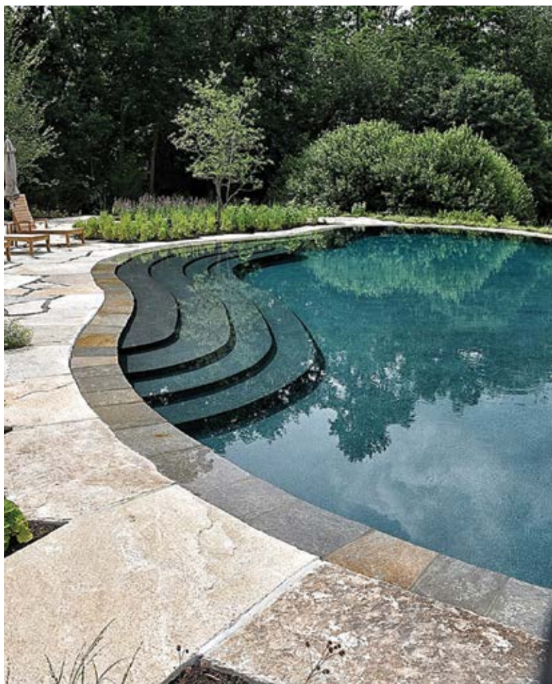
Fig. 4: A free-form pool with a perimeter overflow edge and complex step detail is executed with the shotcrete process
