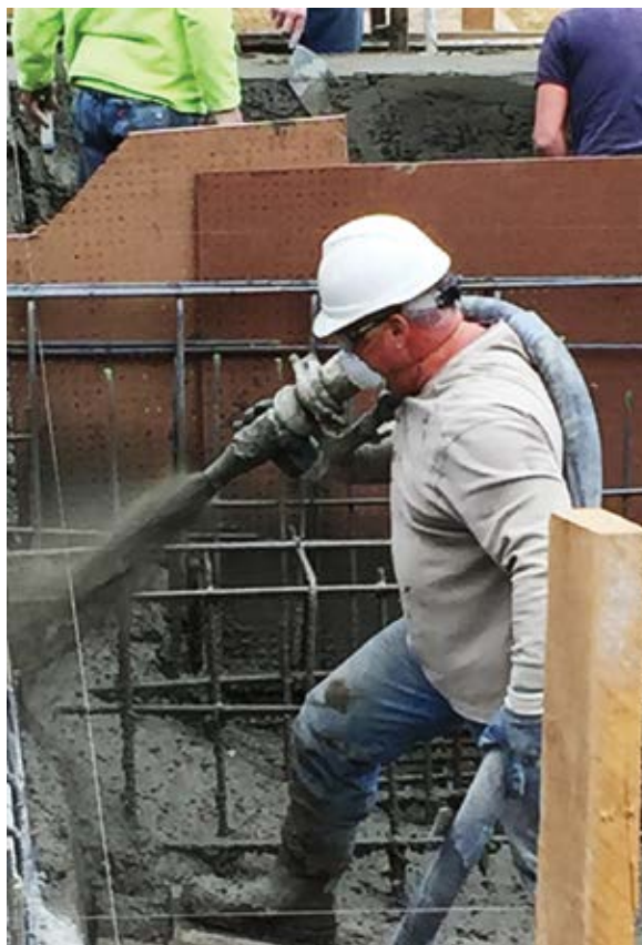
Fig. 2: Nozzlemans work in tandem with other trained crewmembers to ensure a successful application
