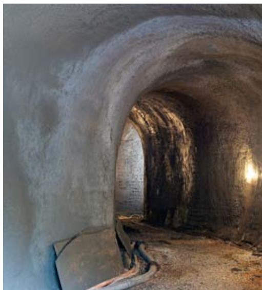
Fig. 5: Organic shape is sculpted wet shotcrete, hand-raked and troweled
