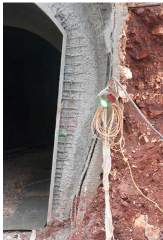
Fig. 2: Dry-mix shotcrete was used for structural support during excavation
