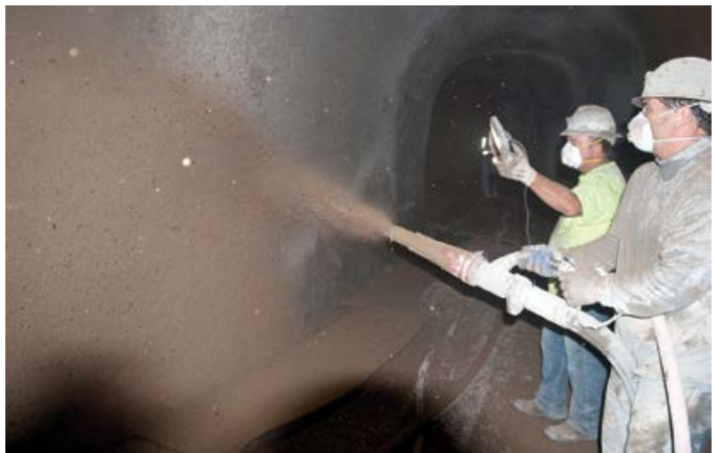
Fig. 4: Wet-mix shotcrete was applied 6 in. (150 mm) thick over welded wire reinforcement in four passes
