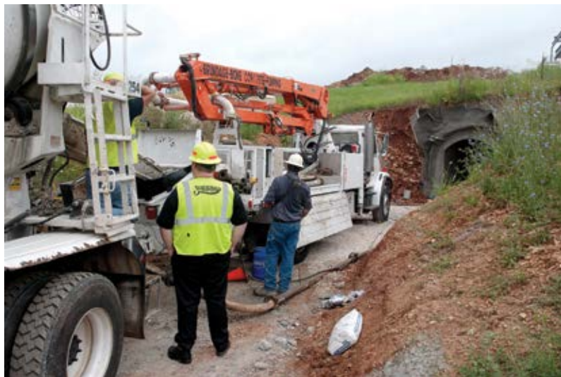
Fig. 6: Schwing S17 with 180-degree discharge serves as line pump for shotcreting up to 400 ft (120 m) inside the tunnel
