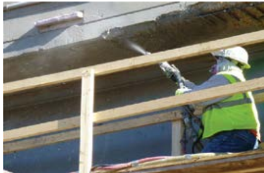
Fig. 2: Shotcrete repair under a bridge
