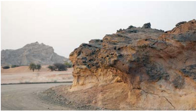
Fig. 4: Artificial rock made by shotcrete in the Al Ain Wildlife Park & Resort, UAE. Winner of the 2011 ASA Outstanding International Shotcrete Project
