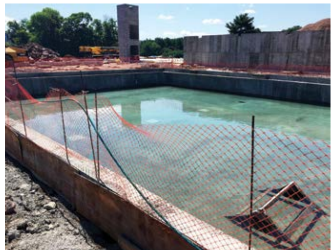
Fig. 3: Watertight tank test
