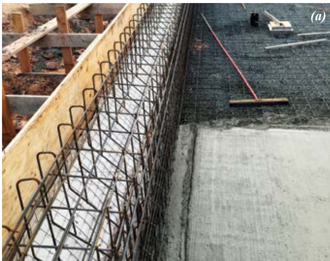
Fig. 1: Floor cast with installed keyway
