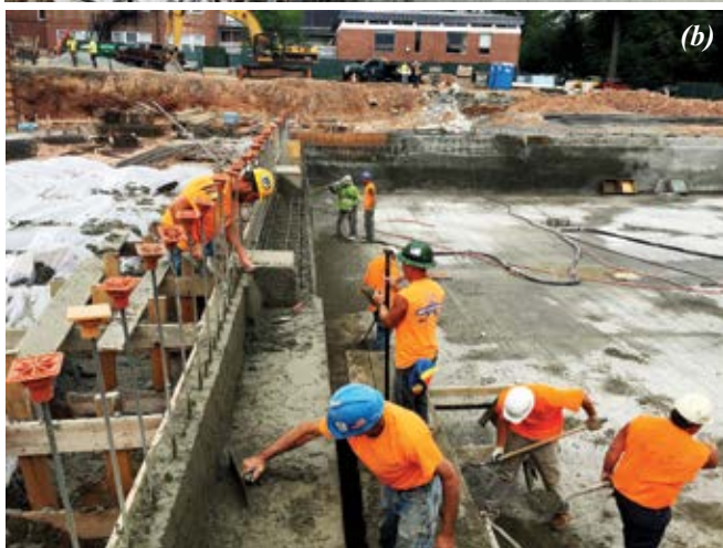
Fig. 2(a) and (b): Shotcrete on top of cast floor
