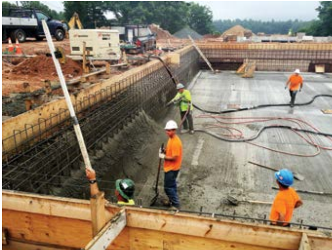
Fig. 1: Floor cast with installed keyway
