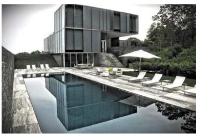
Shotcrete makes up the body of this radiant, glass-like Lautner-edge project. In addition, it was used to create the full-perimeter surge trough into which the pool's water flows
