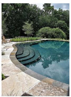
With careful forming, properly executed shotcrete can create tight tolerances for free form stairs that are comparable to those that can be achieved by cast-in-place concrete. In this case, that execution was a key component of this nature-inspired slot-overflow pool
