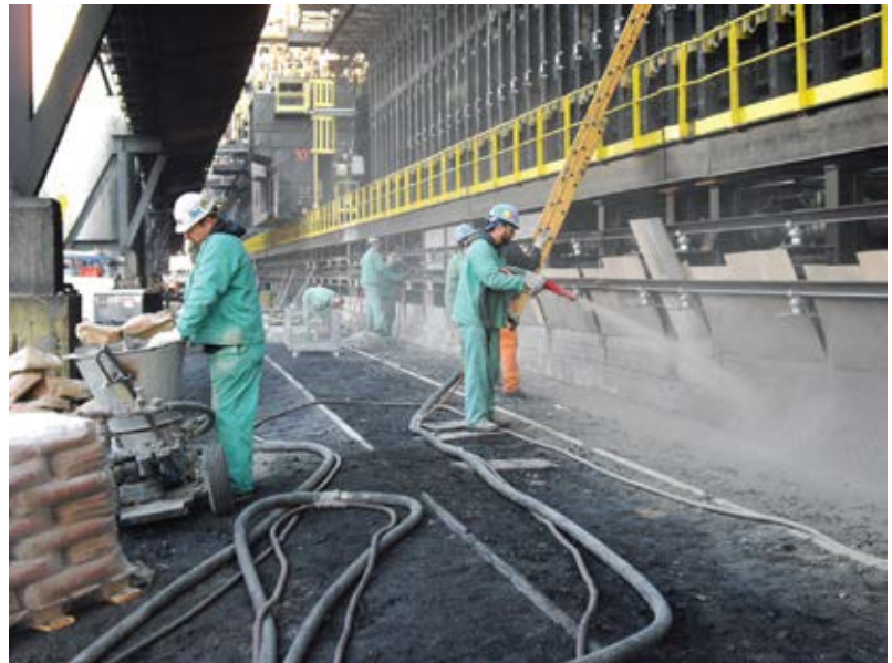
Fig. 3: Modern dry-mix shotcreting
