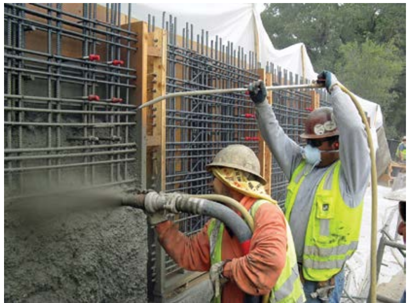
Fig. 4: Wet-mix shotcreting of structural wall
