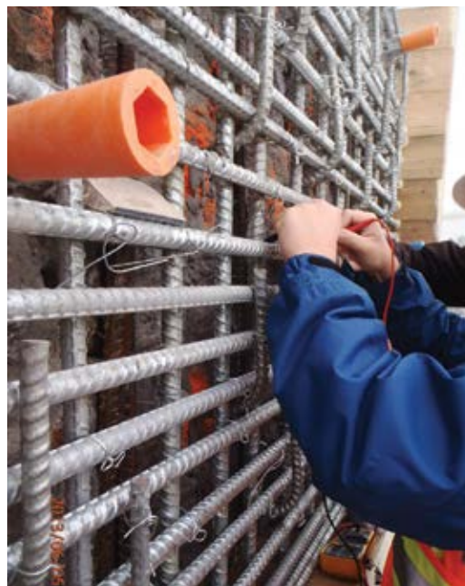
Fig. 3: Reinforcing bar sentinel tie-in
