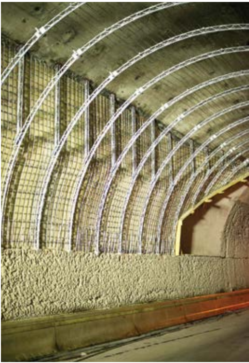
Fig. 8 (left and above): Construction sequence Step 3—lattice girder and extrados reinforcement sidewall sections
