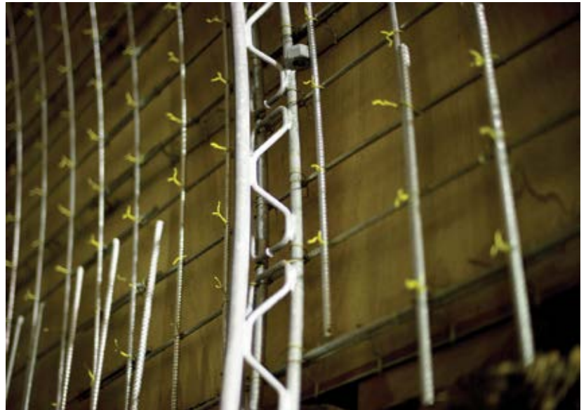
Fig. 8 (left and above): Construction sequence Step 3—lattice girder and extrados reinforcement sidewall sections
