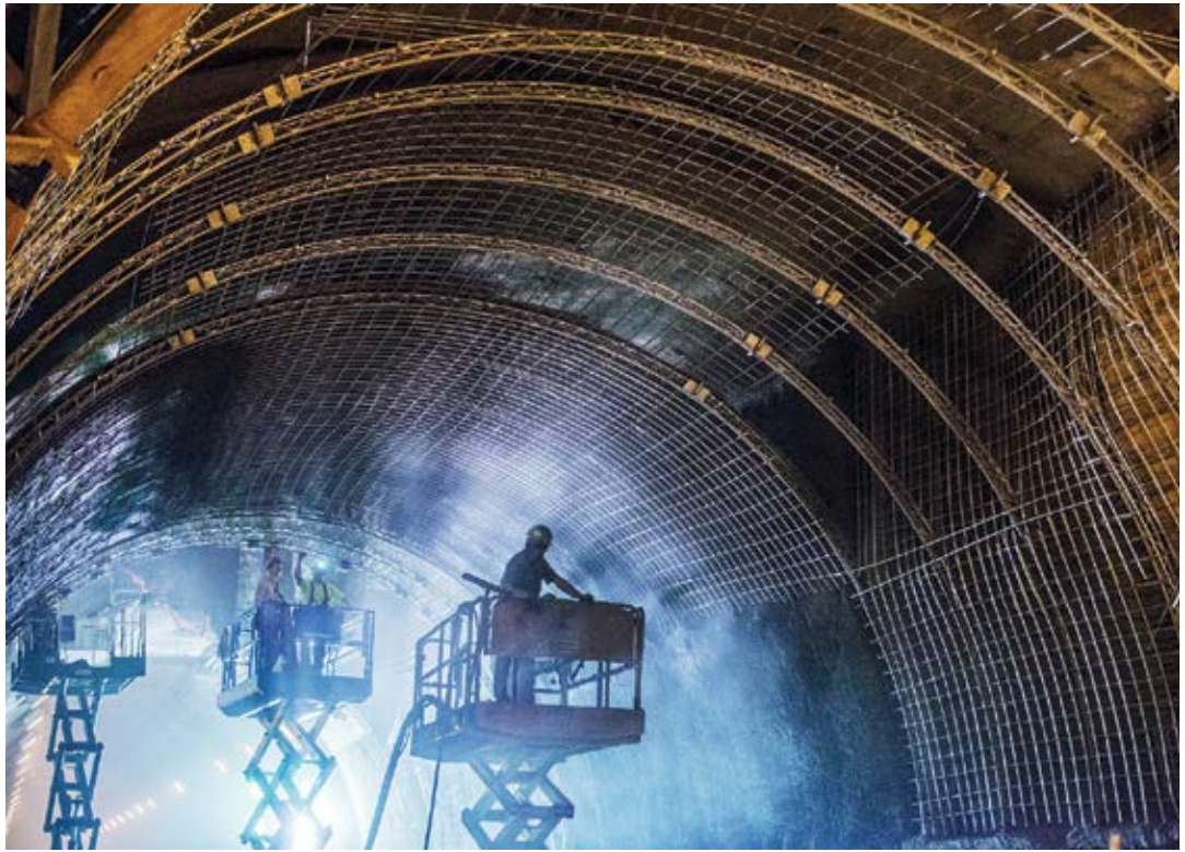
Fig. 10: Construction sequence Step 5—preparation of center arch section
