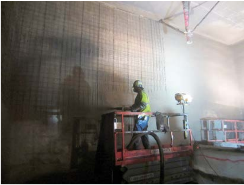
Fig. 4: Shotcrete placement
