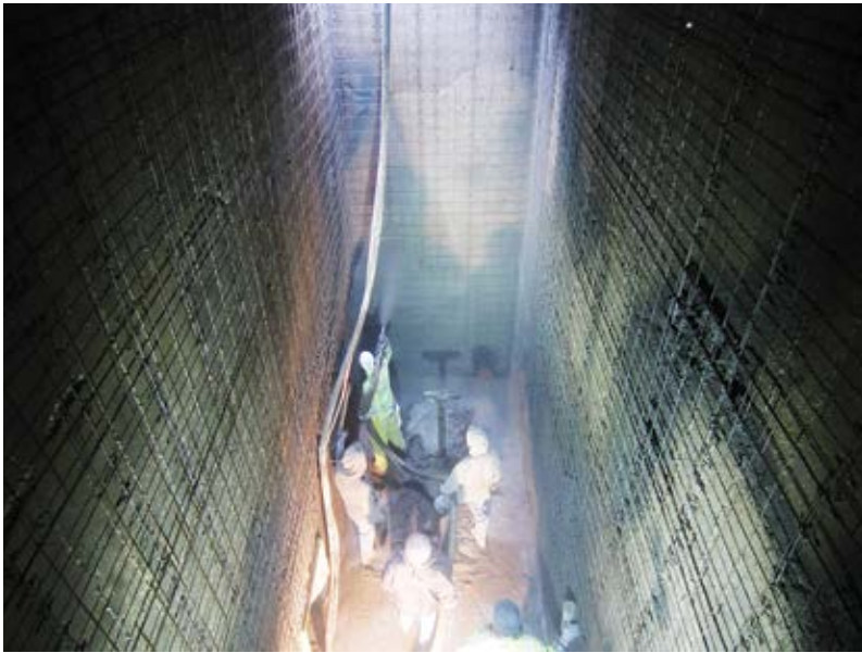
Fig. 5: Shotcrete placement at weir
