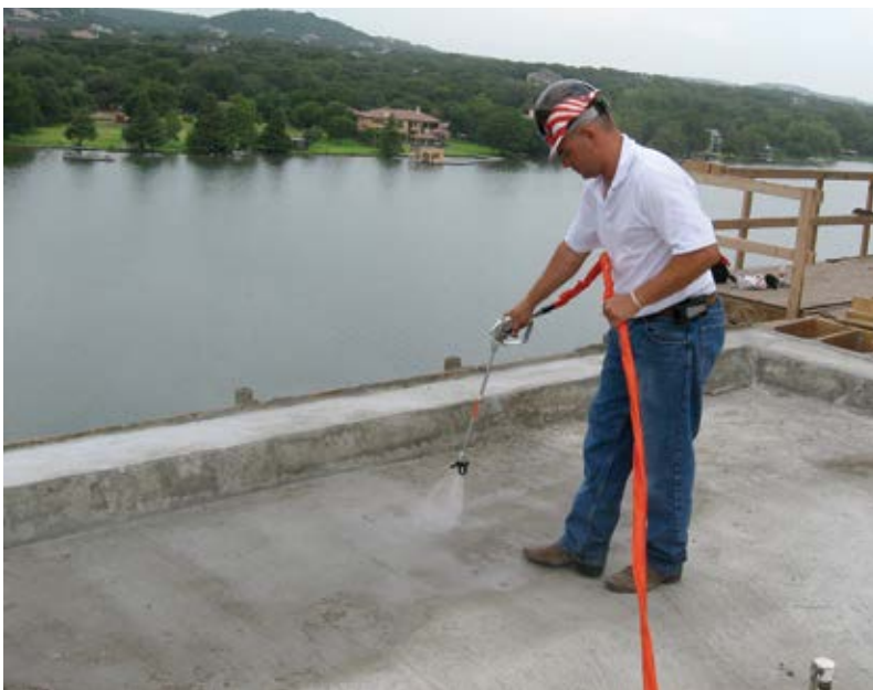
Fig. 6: Example of spray-applied densifier
