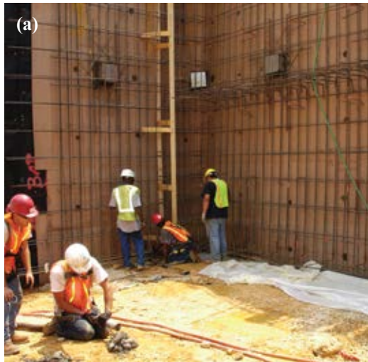
Fig. 2: (a) The corner of this photo was the starting point for shotcreting; and (b) one of the biggest challenges faced was the wall reinforcing steel moving out 4 in. (100 mm) by the weight of the shotcrete
