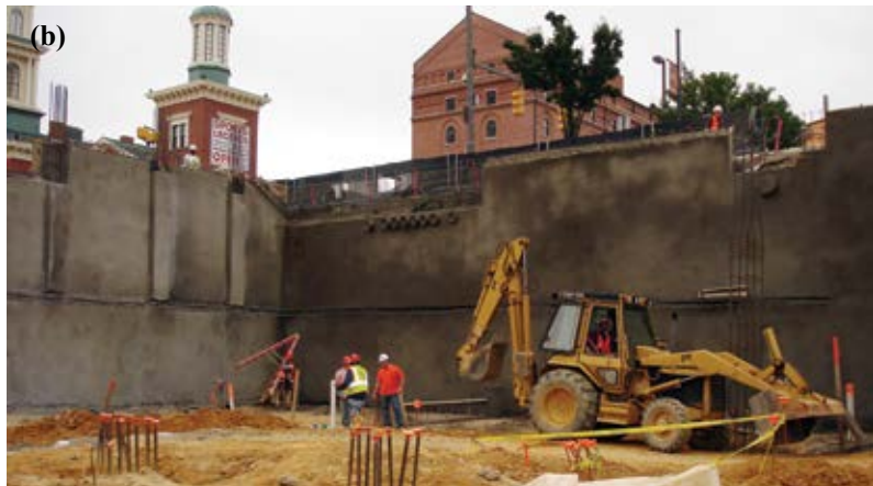
Fig. 9(a) and (b): Finished wall with the floor waterproofing being installed, and the same wall after it was finished
