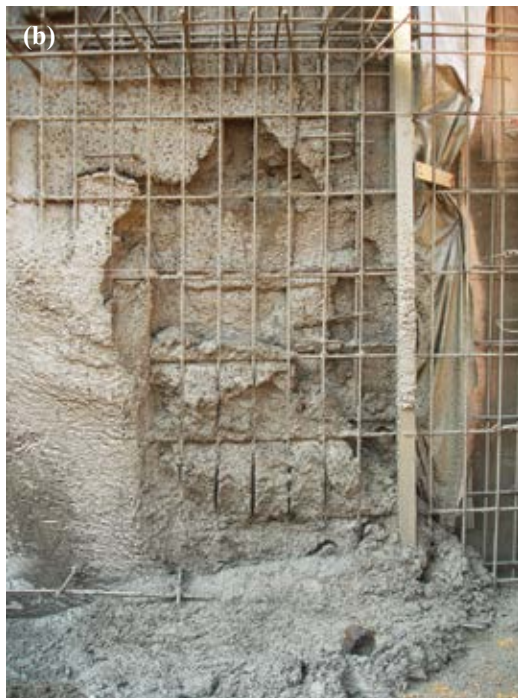
Fig. 2: (a) The corner of this photo was the starting point for shotcreting; and (b) one of the biggest challenges faced was the wall reinforcing steel moving out 4 in. (100 mm) by the weight of the shotcrete
