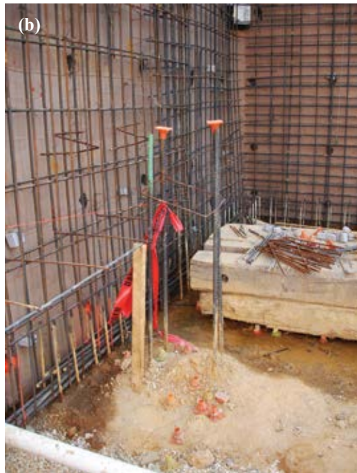
Fig. 5(a) and 5(b): Congestion in front of the next wall sections to be shot
