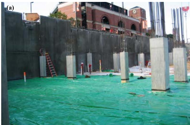
Fig. 9(a) and (b): Finished wall with the floor waterproofing being installed, and the same wall after it was finished
