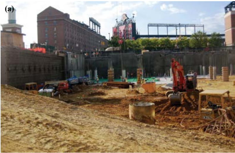
Fig. 5(a) and 5(b): Congestion in front of the next wall sections to be shot
