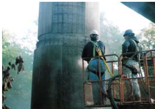
With good surface preparation and gunning practices, shotcrete provides an excellent bond to the existing substrate
