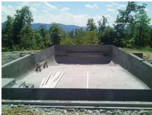
Fig. 4: Pool shell complete before tile and coping installation
