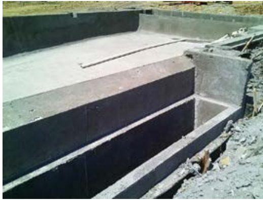
Fig. 3: Catch basin for vanishing edge before finishes
