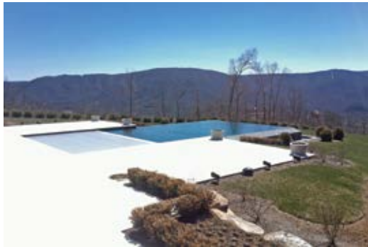
Fig. 5: Floating automatic cover being retracted into hidden cover housing
