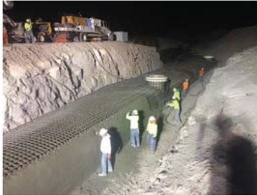
*Fig. 1: Nighttime shotcrete placement*
