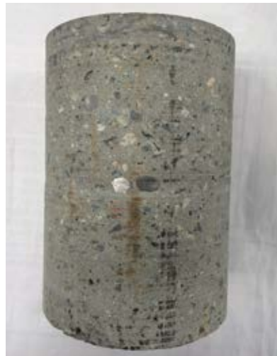
Fig. 3: A core sample from the pool wall where layering was done. Shows excellent reinforcing bar encapsulation and no actual layers
