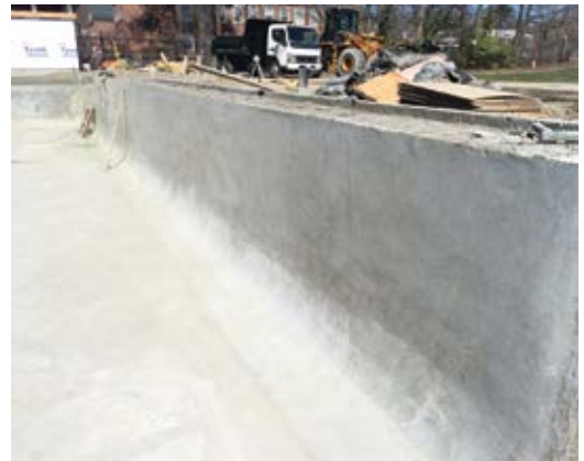
Fig. 5: The steel troweled final finish
