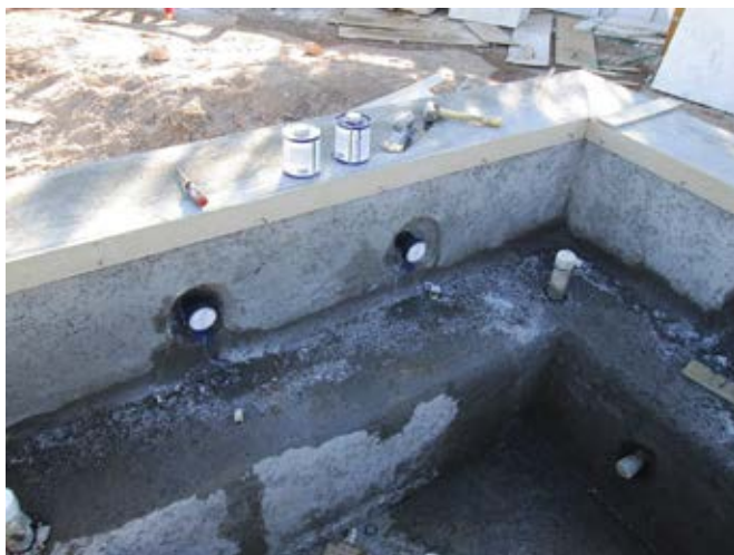
Fig. 2: Piping with and without fitting prior to sealing
