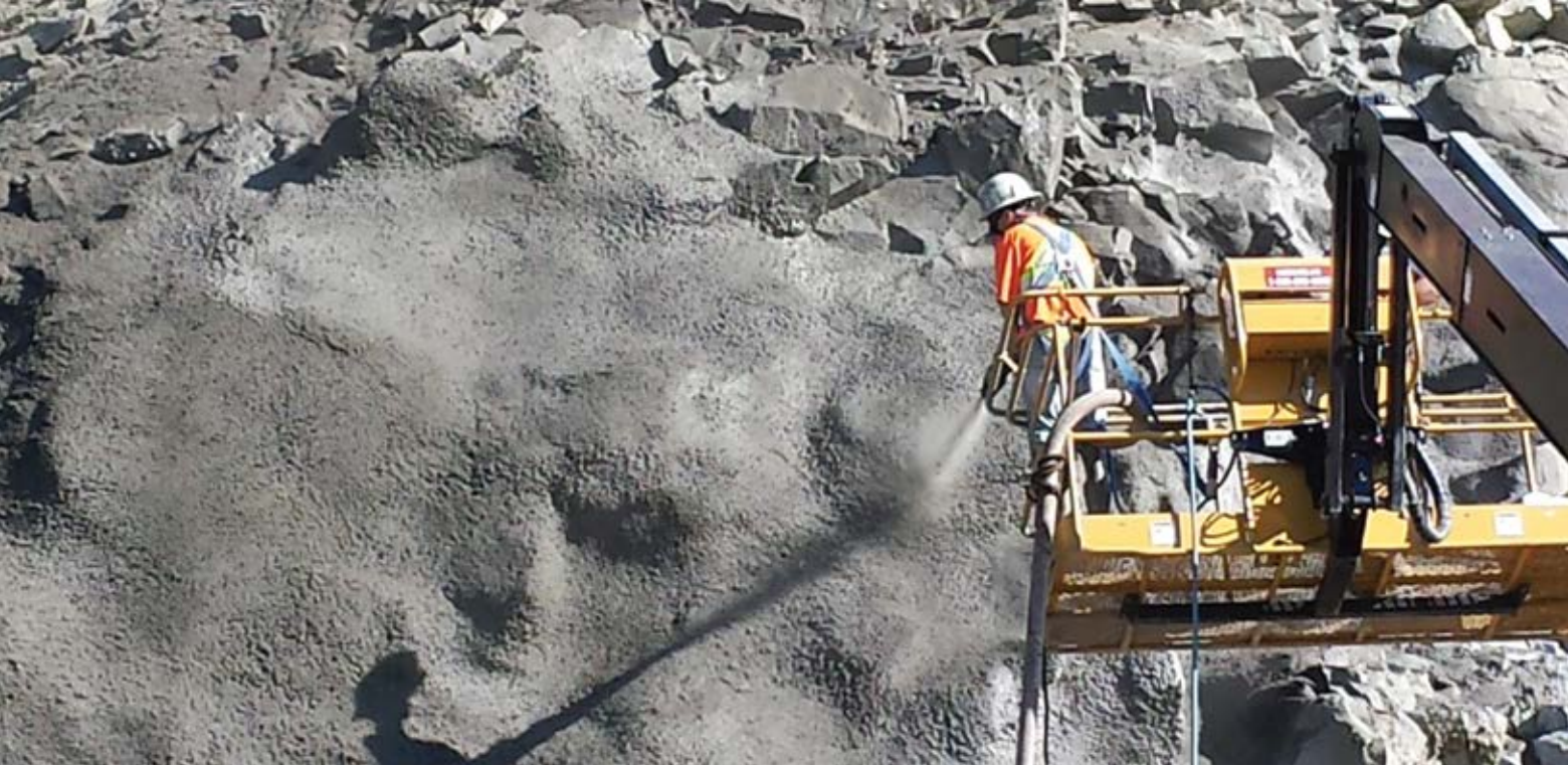
Fig. 1: Steel fiber-reinforced dry-mix shotcrete
