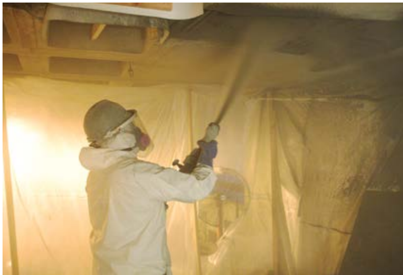
Fig. 1: Dry-mix shotcrete nozzleman using predampened materials during a parking garage repair
