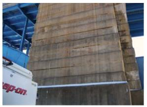
Fig. 1(a): Dry-process shotcrete repairs on 31st Street Bridge in Pittsburgh, PA, were done in 1973 over bottom two-thirds of this pier. Architectural details were maintained and shotcrete repairs remain in good condition 42 years after they were installed
