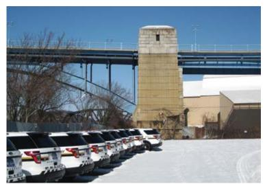
Fig. 1(b): This pier on Pittsburgh side of Allegheny River required extensive repairs and shotcrete also remains in very good condition
