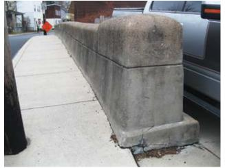
Fig. 2(b): Concrete on both sides of parapets under capstones were badly deteriorated. They were chipped out then replaced with dry-process shotcrete 38 years ago
