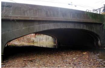
Fig. 2(a): Arches and parapets of this single-arch bridge in Bridgeville, PA, were badly deteriorated before shotcrete repairs in 1977. Dowels and reinforcing bars were installed and dryprocess shotcrete placed across arches on both sides of bridge
