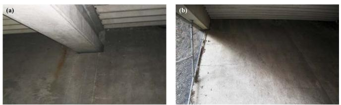
Fig. 6 (a) and (b): (After) Dry-process shotcrete was used to stabilize slope for parking garage that was built into hillside behind Carnegie Museum in 1988. These photos of that work taken in February 2015 (27 years later) show that work remains in good condition. Sections of shotcrete slope can be seen on each level of parking garage
