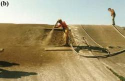
Fig. 3(a) and (b): (Before) Rehabilitation work on Raccoon Dam and Spillway (Raccoon State Park, PA) included removal and replacement of deteriorated concrete on large sections of spillway and across top of dam. These photos show dry-process shotcrete placed on upper sections of dam in autumn of 1984. Once placed, shotcrete was then cut down or rodded to grade before finishing
