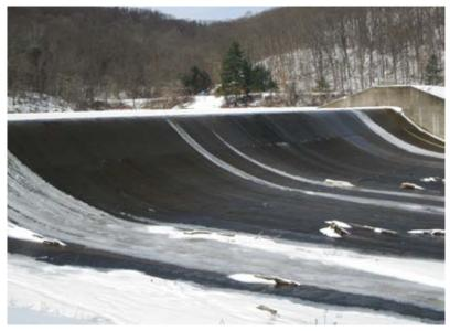
Fig. 4: (After) Shotcrete repairs to Raccoon Dam remain in good condition across crest of dam 31 years after shotcrete work was performed. Water flowing over crest of dam and spillway shows a relatively even flow despite the passage of years
