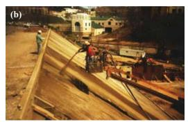
Fig. 5(a) and (b): (Before) In 1988, dry-process shotcrete was placed for slope stabilization on hillside behind Carnegie Museum in Pittsburgh, PA. Recesses were left for precast concrete to support a parking garage that was later built over the hillside
