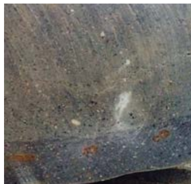
Fig. 8(b): Arch cut, two layers
