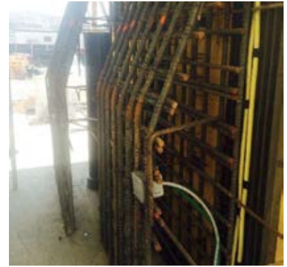
Fig. 6(c): Wall mockup in single pass
