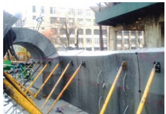
Fig. 8(c): Cut mockup
