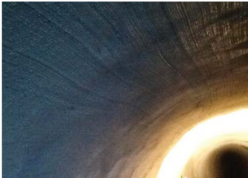
Fig. 7: Finished shotcrete lining
