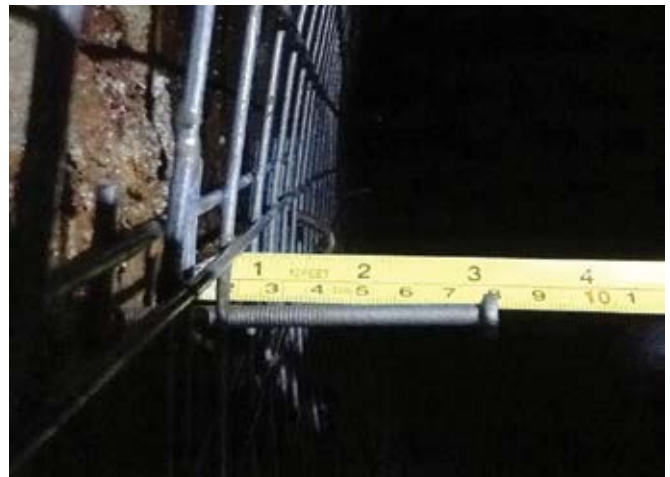
Fig. 5: Measuring pin installed to ensure correct thickness of shotcrete
