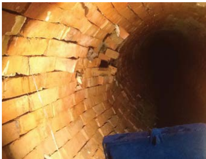
Fig. 1: Existing 100-year-old brick combined sewer
