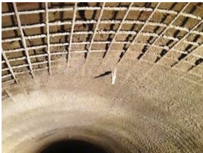
Fig. 4: First lift of dry-mix shotcrete
