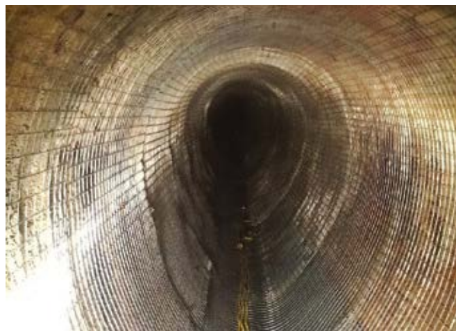
Fig. 2: Installed galvanized welded wire reinforcement (2 x 2 in. [50 x 50 mm], 12 gauge)
