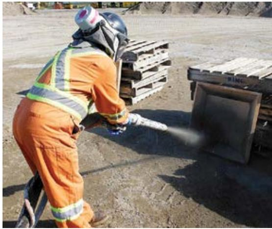
Fig. 3: Nozzleman shooting a test panel for later-age strengths and durability properties
