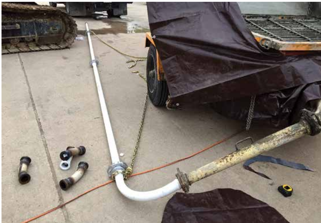
Fig. 2: A great example of a thrust chain setup
