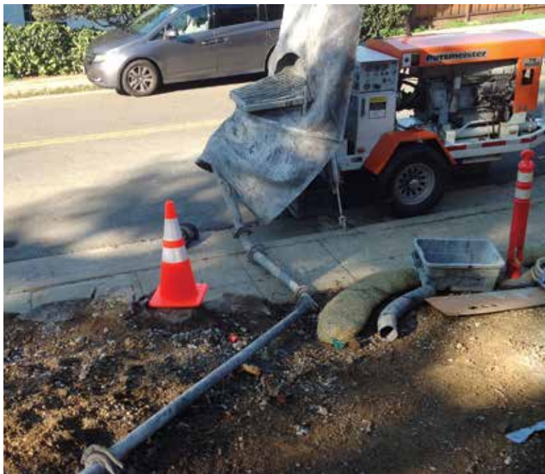
Fig. 1: A few pieces of metal pipe can greatly improve work station safety
