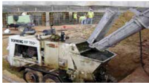
Fig. 14: Schwing 750 trailer pump setup for easy maneuvering in and around the jobsite can be reduced down to a 2 in. (50 mm) hose for shotcrete work or up to 5 in. (125 mm) for concrete pumping
