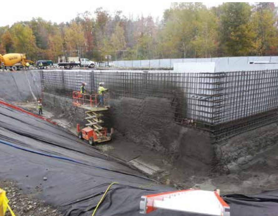
Fig. 3: Using the lift on the research tank allowed us to easily reach the 20 ft (6 m) heights and move along quickly and safely
