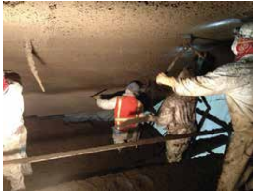
Fig. 8: Cutting of guides and finishing
