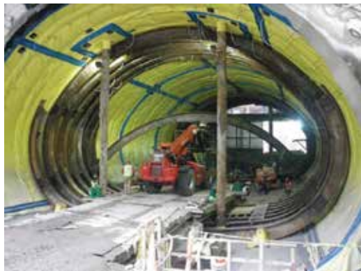
Fig. 4: Waterproofing and ring girders being installed
