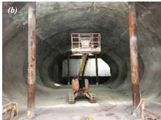
Fig. 9: Finished tunnel looking east to west under Northern Boulevard
