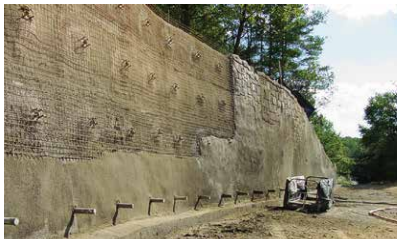
Fig. 2: Top wall being transformed with faux-rock finish
