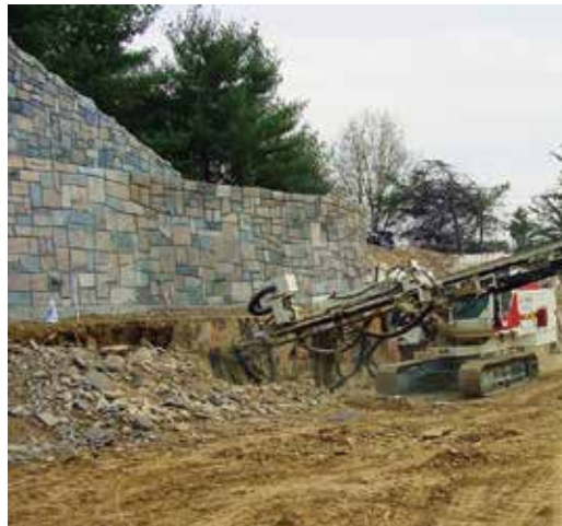
Fig. 5: Soil nailing
