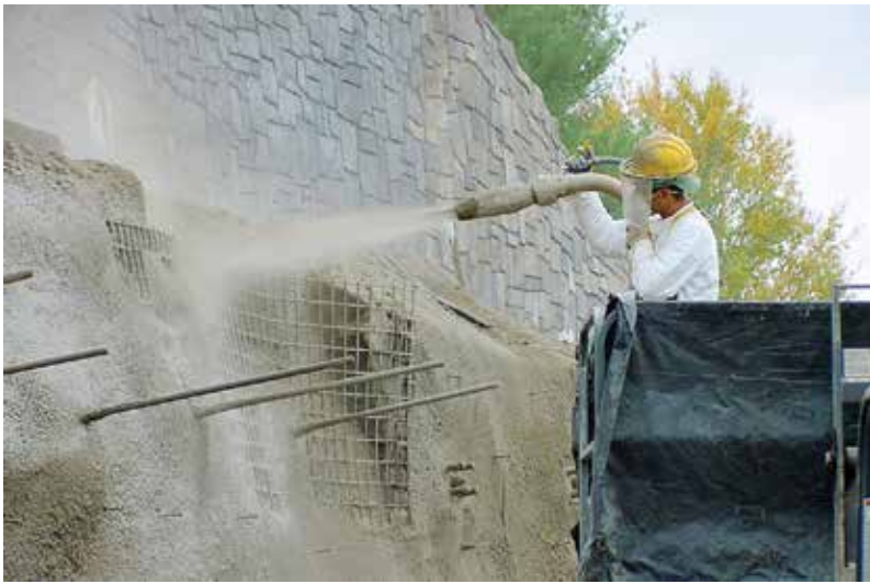
Fig. 6: Shotcrete placement
