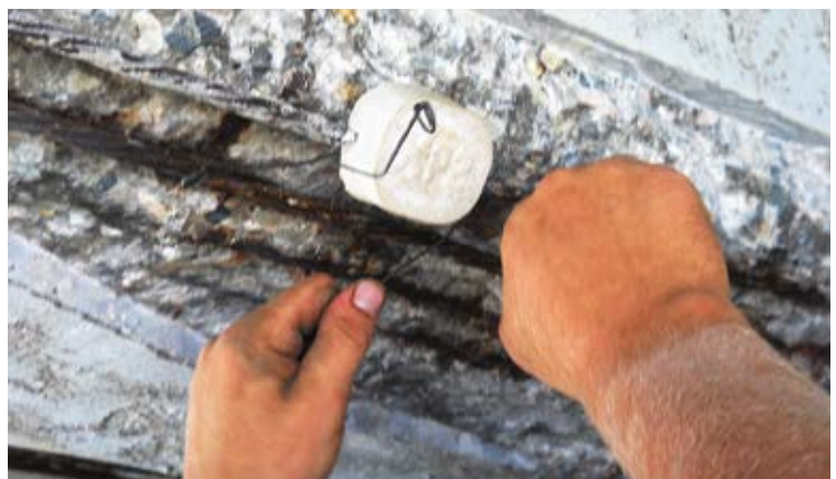
Fig. 3: Galvanic anode for concrete repair
