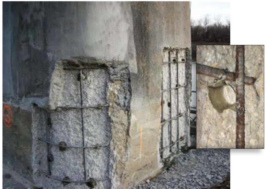
Fig. 5: Embedding mortar used to create a conductive path between the anode and the concrete substrate
