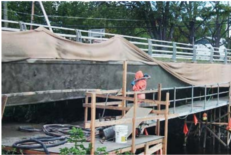
Fig. 7: Type 2 anode repairs completed with dry spray shotcrete
