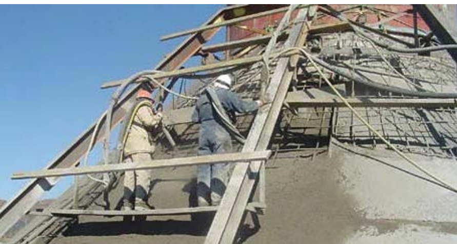
Nozzlemen shooting the base of the lighthouse
