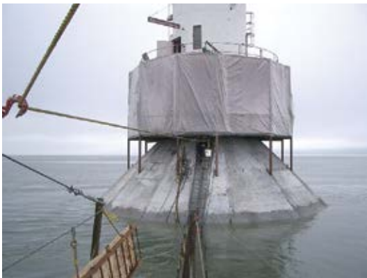
Completed shotcrete application at low tide
