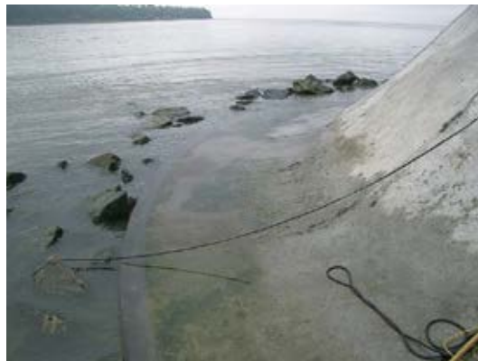
Completed shotcrete application at low tide
