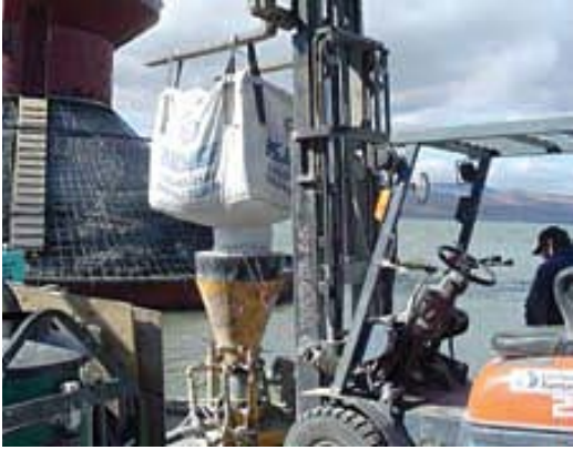
Shotcrete was supplied in 2200 lb (1000 kg) reusable, bulk tote bags
