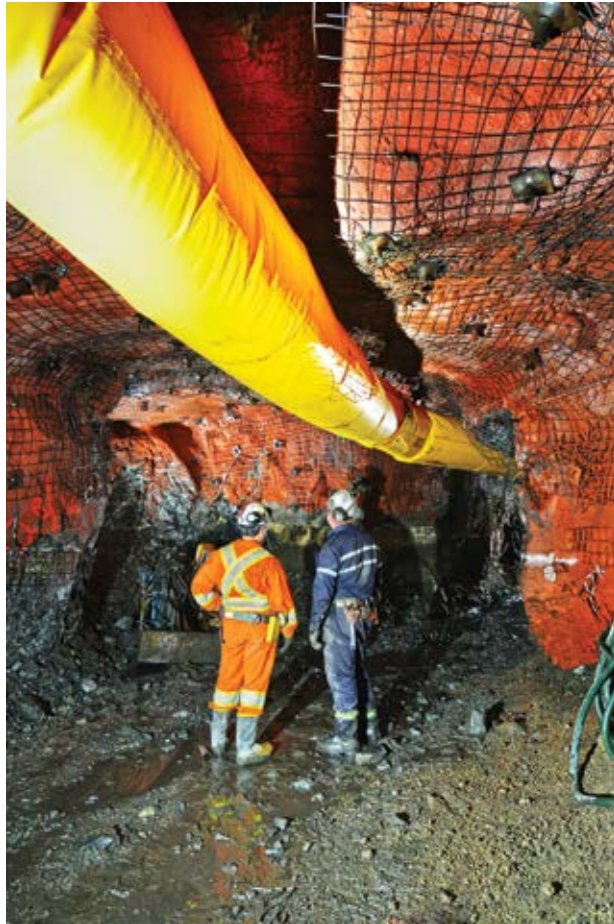
Fig. 2: Shotcrete mixtures using new cement technology that achieve compressive strengths as high as 2900 psi (20 MPa) after only 2 hours have recently been introduced to the mining and tunneling industries
