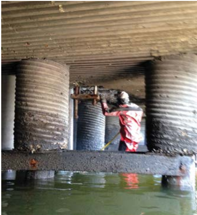
Fig. 5: Unsound concrete removed with pneumatic chipping hammers
