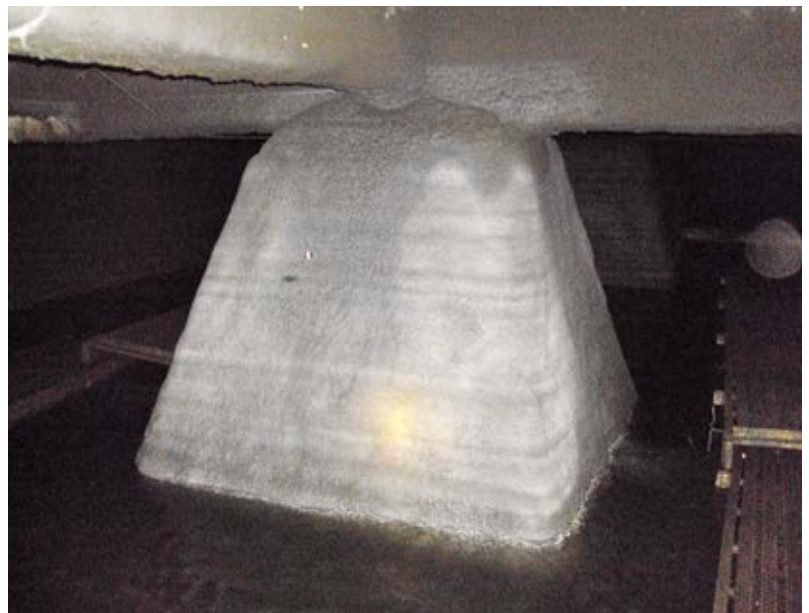
Fig. 4: Triangle-shaped piles and underdeck beams repaired and encased with shotcrete
