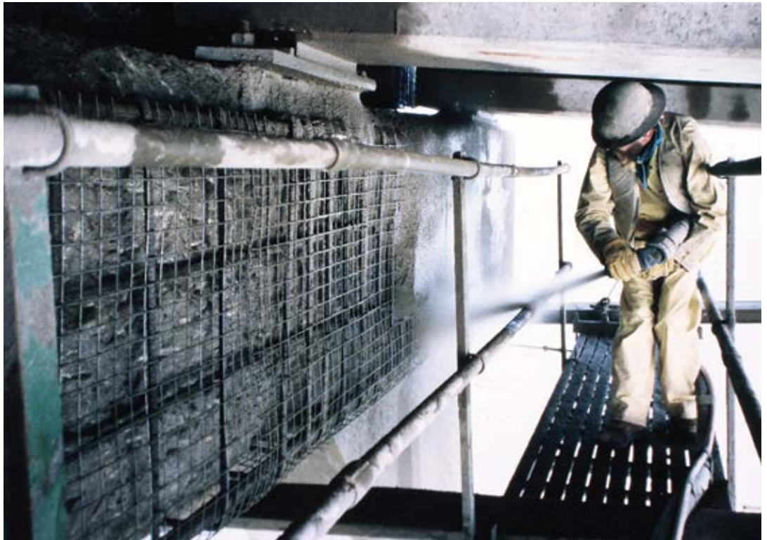
Fig. 5: Shotcreting pier cap
