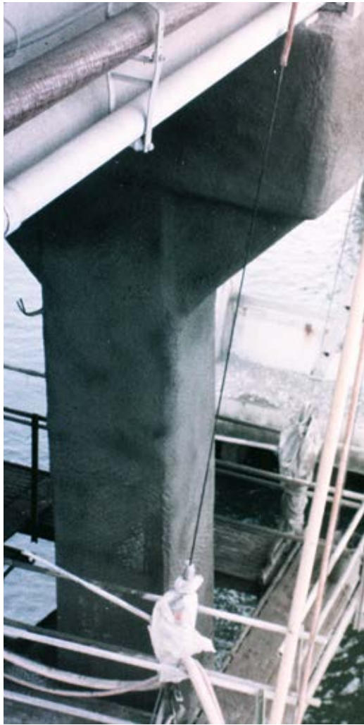
Fig. 4: Freshly shot pier column
