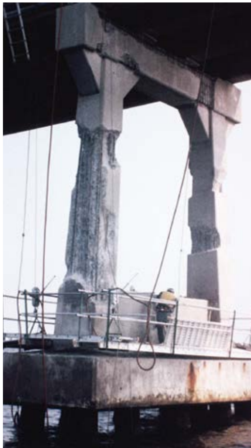
Fig. 3: Unsound concrete removed
