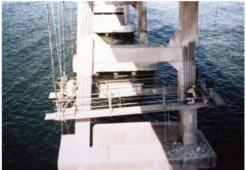
Fig. 2: Chipping of unsound concrete
