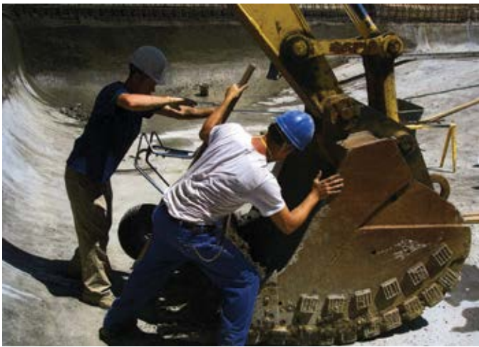
In this case, the pool was so deep that an excavator was kept on hand to ease removal of any concrete spoils or incidental rebound. Frequent tests were also conducted to make certain the shotcrete material was being applied at (or beyond) the specified strength
