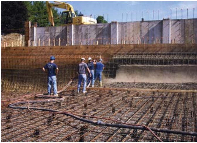
Delivering on the commitments made to the design team was largely a matter of following usual procedures for shotcrete application, including construction of solid, non-vibrating forms; installation of reinforcing steel to ensure complete concrete coverage; and a systematic, patterned approach to what was to be a multi-day shoot
